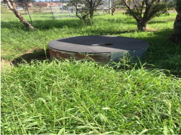
Photo 7. Septic tank identified at the rear of the post office
