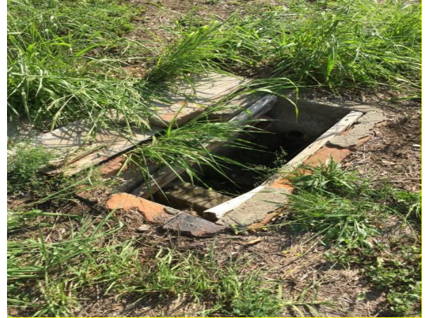
Photo 8. Brick pit located at the rear of the post office
