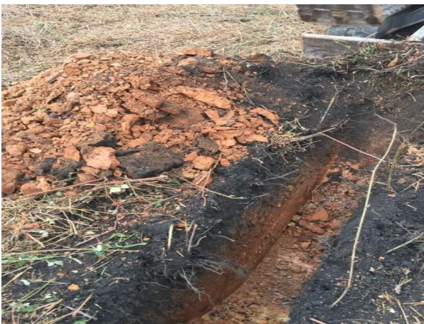
Photo 11. Black discoloured soils were noted at TP7
